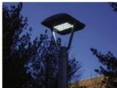
Figure 1. Several HPS fixtures (left) were replaced with LED pole-top mounted luminaires (right) to illuminate a pedestrian area at a Federal Aviation Administration facility in Atlantic City, NJ. A full report on this installation is available at [www.nerl.doe.gov/ssl](http://www.nerl.doe.gov/ssl).
